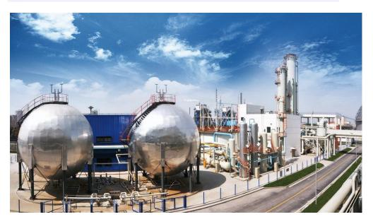
In 2009, world's largest CO<sub>2</sub> capturing facility, with capturing capacity of 120,000 t/a, was put into operation in Huaneng Shanghai Shidongkou Power Plant.
