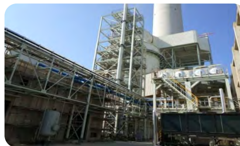
Nov 2018, steel structure of the amine device 90% completed; compression and purification device installed
