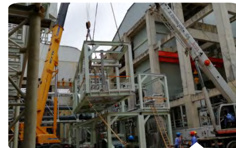
Nov 2018, membrane device installation
