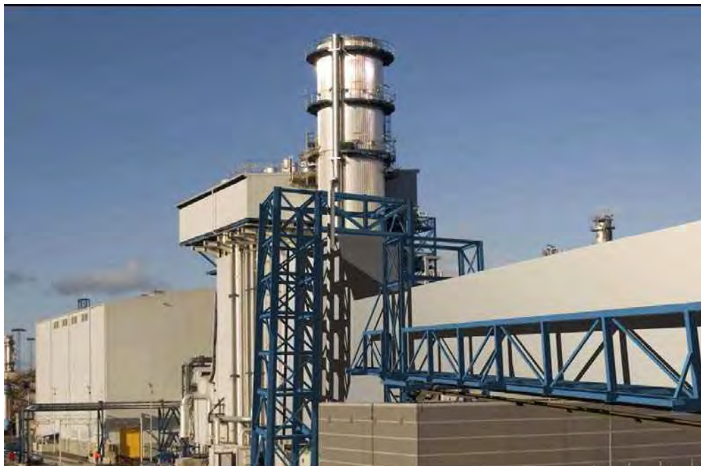
Figure 3-1. HRSG Stack Modification with Duct Work
